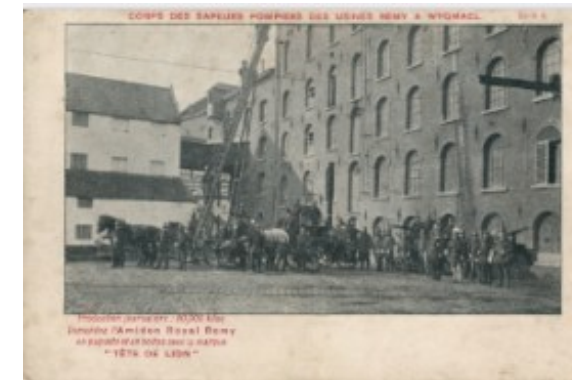
The factory had a significant firefighting crew.
